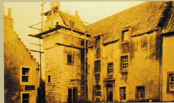
Restoration in progress at Culross: left, Sandhaven area; above, the Study
