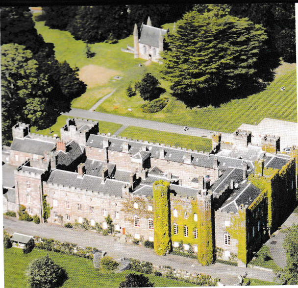
Aerial view of Scone Palace showing the Chapel on Moot Hill.
